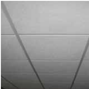
Suspended T-bar & ceiling tiles (min. 8 mm)
